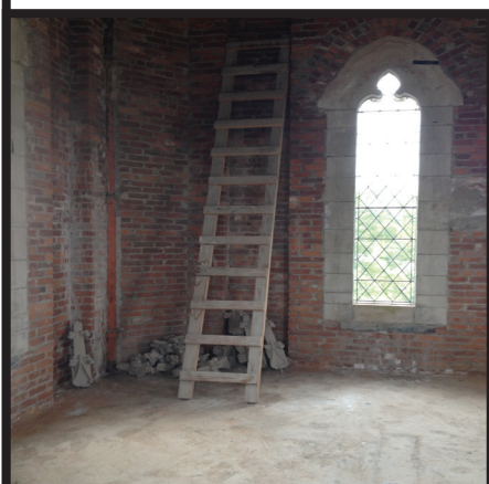
View from inside the third floor of the Starr Hall Tower
